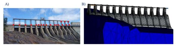
Figure 8: A) Studied spillway and location of measurements(•); B) Numerical model
